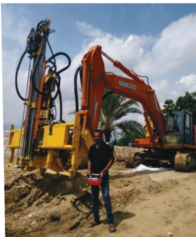
Testing done at site - Tiruchengode, Tamil Nadu
