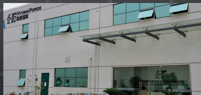
Asian/Pacific headquarters, precision machining and manifold assembly facility in Changzhou, China, near Shanghai.
