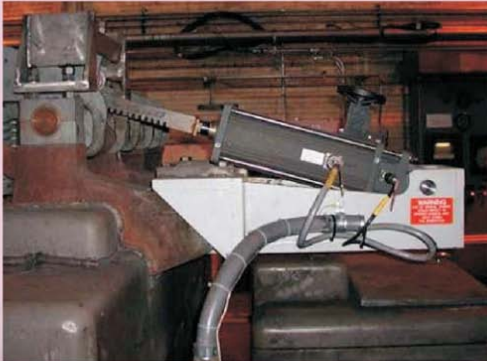
Steam Turbine Retrofit
